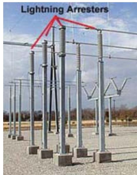
Lightning arresters on bus structures
