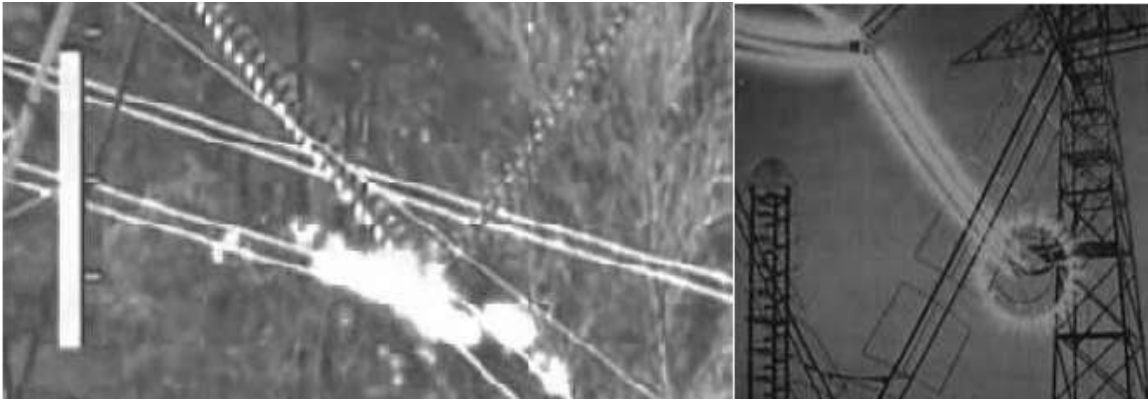
Figure 2: Images of Corona in High Voltage Transmission Lines
