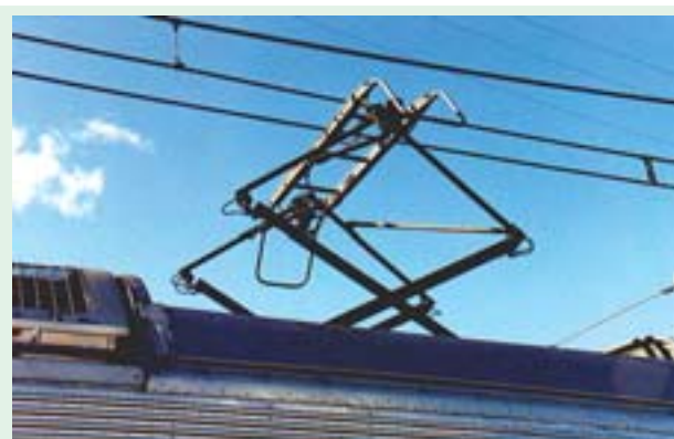
The pantograph mechanism helps to maintain a link between the overhead contact wire and power circuit of the electric locomotive
