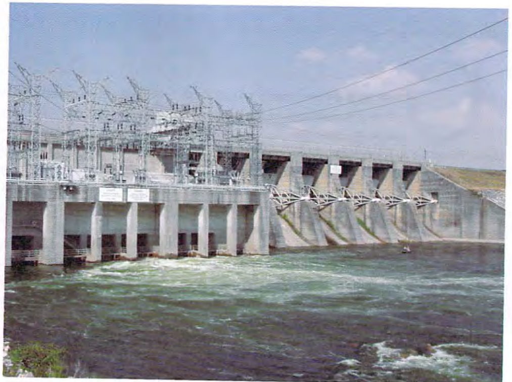
Figure 11.1 → Hydroelectric generating facility. (Courtesy of Mark Nelms)
